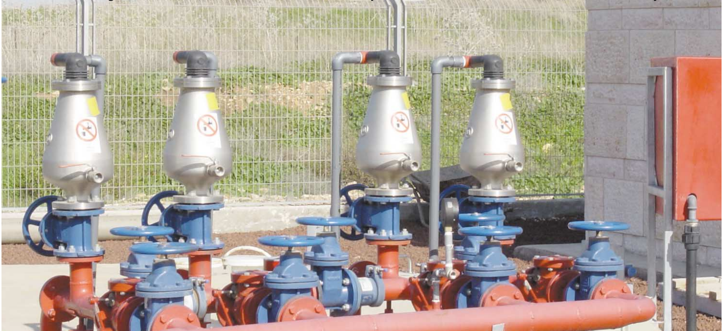
Sewage pumping station “Hefer” project
